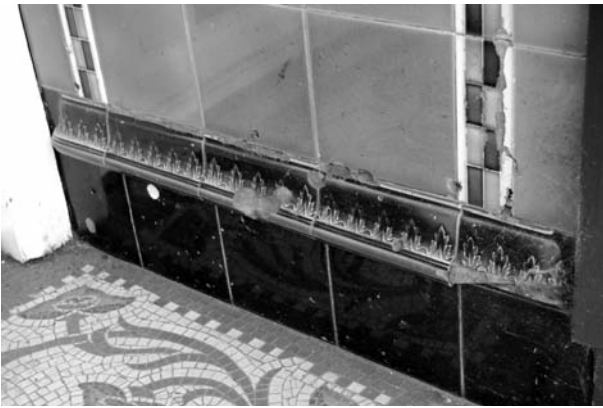
Figure 12. Lobby panel at 138 High Street, Dunbar before conservation
