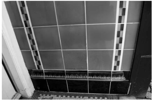
Figure 13. Lobby panel at 138 High Street, Dunbar after restoration using Craven Dunnill tiles
