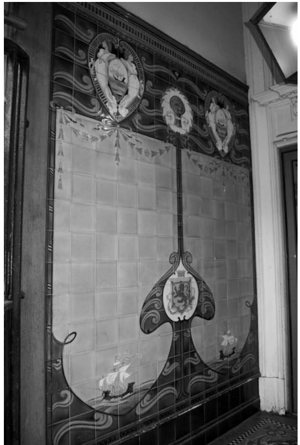
Figure 11. Part of tile scheme at former Paisley Provident Co-operative Society
